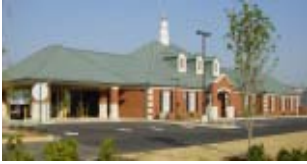
Heritage Bank is located in Fayetteville, Georgia. Group VI has constructed 11 banks in the Metro Atlanta area.
