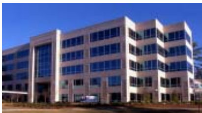
The IRS has leased the majority of this Group VI Building at 6655 Peachtree Dunwoody Road in Atlanta, Georgia
