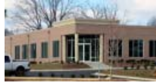
Marena Group's new 12,000 square foot manufacturing and distribution headquarters is located in Lawrenceville, Georgia.
