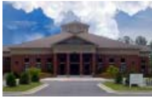
Group VI completed the 28,000 square foot Sunrise Baptist Church of Lawrenceville, Georgia in July 2002.
