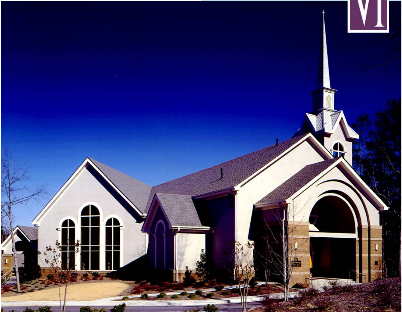
First Presbyterian Church of Peachtree City Peachtree City, Georgia Architect: Foley Design Associates
